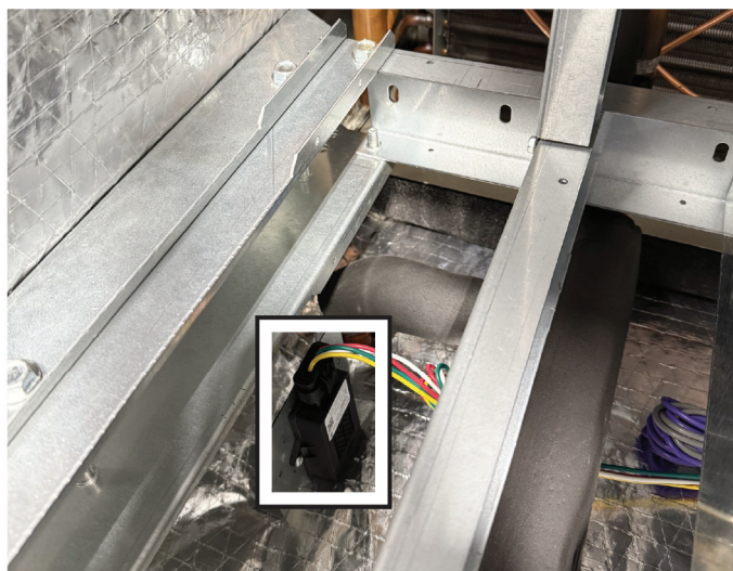
Figure 21: RDS Sensor Installation
