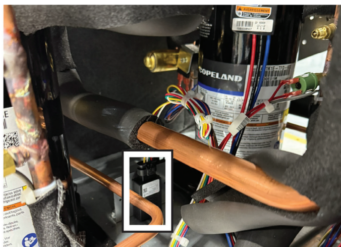
Figure 21: RDS Sensor Installation
