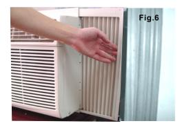
**3** Extend the side panels out against the window frame (Fig.6).
